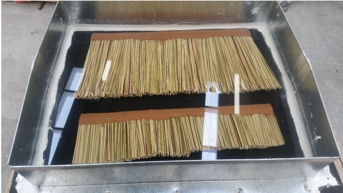
Figure 1: Steel perimeter bund fitted to form a tray over the membrane
